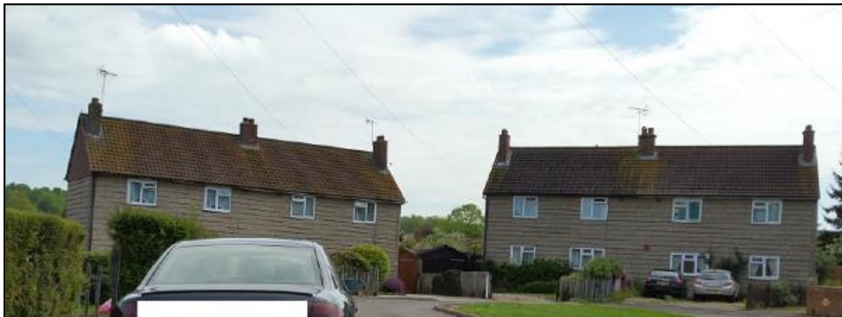
Figure 2 - existing elevational treatments
